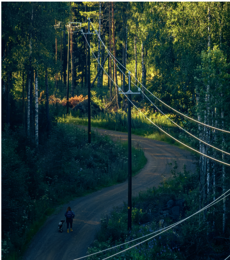
Above: Tanasote treated utility poles
